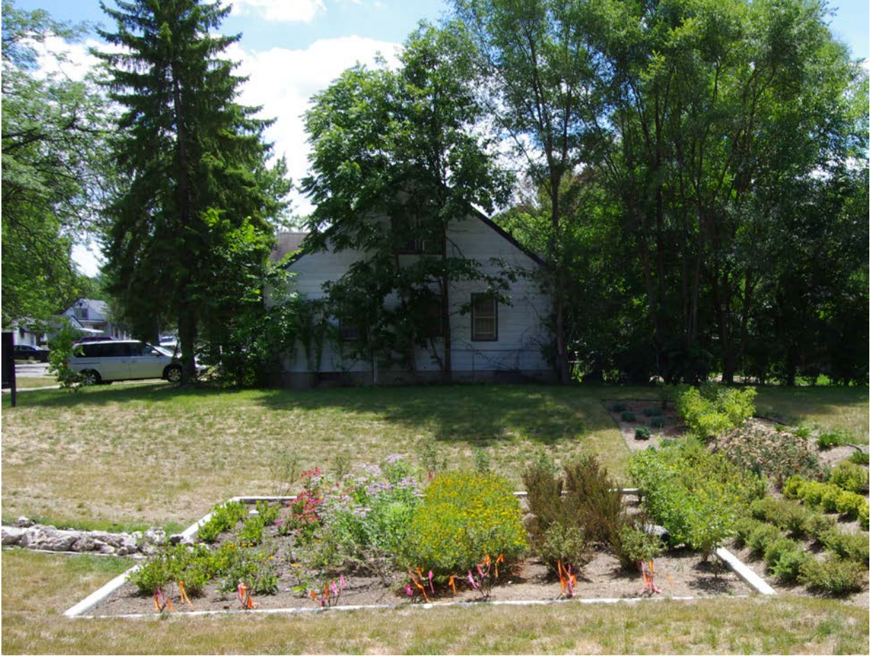
Figure 18. All design alternatives used plants in rows and the crisp edge of a concrete curb around the bioretention area as cues to care.
