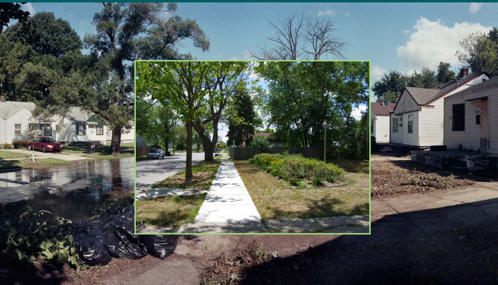
Figure 2. In 2015, we implemented pilot garden designs on four sites in the Warrendale neighborhood of Detroit to relieve stormwater management problems.
