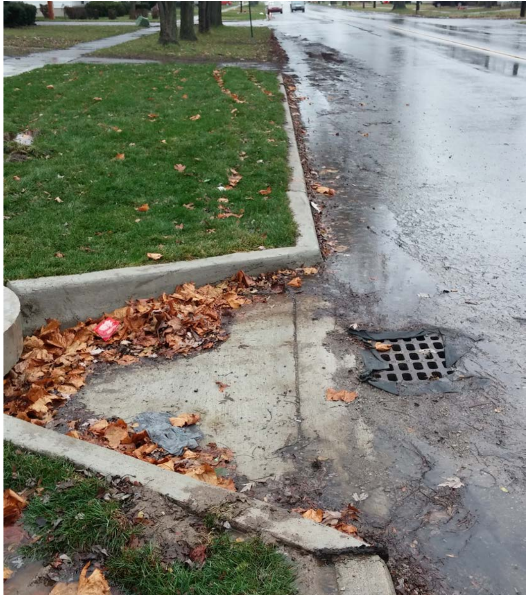
Figure 11. NEW-GI GSI pilot sites capture street runoff. It is considered optimal to place GSI where large amounts of stormwater flow are generated – like streets and parking lots.
